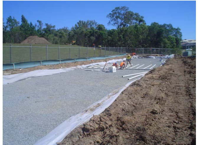
Drainage for the bio-retention basin
