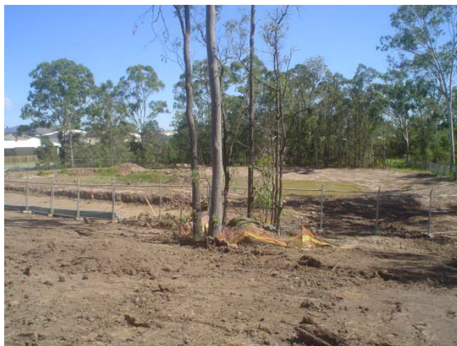
Looking down at the pond
