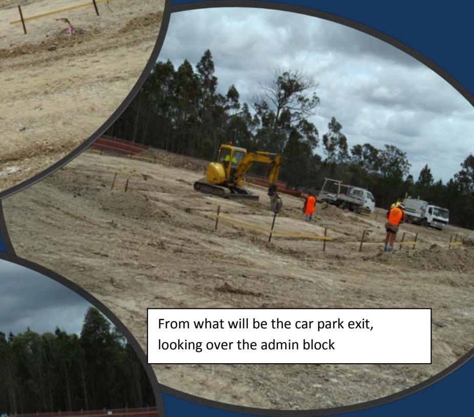
Looking south over the new Prep rooms.....
