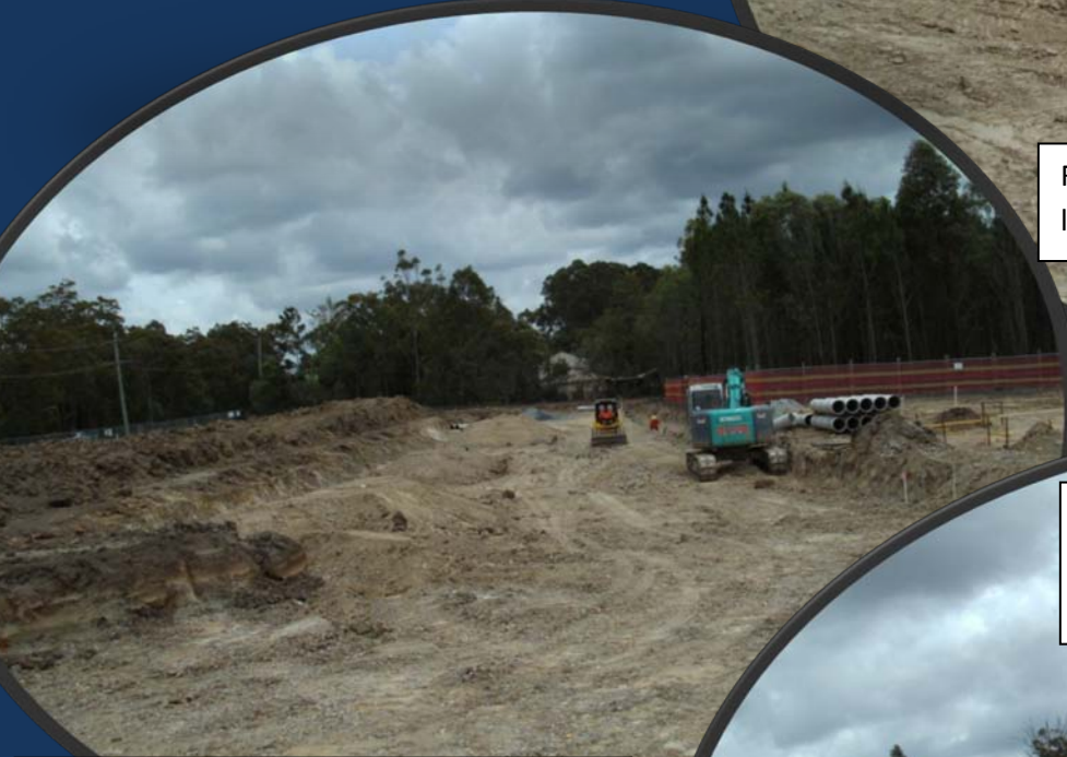
Looking south over the car park. After the stormwater drainage has been completed, the car park will be built back up to surrounding ground level.
